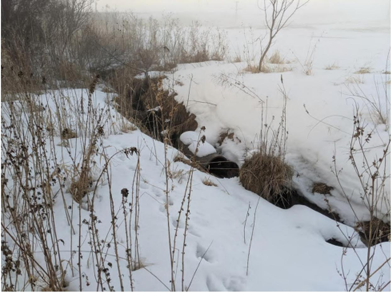
*Figure 1: 1922 Main completely exposed and broken above outlet.*
