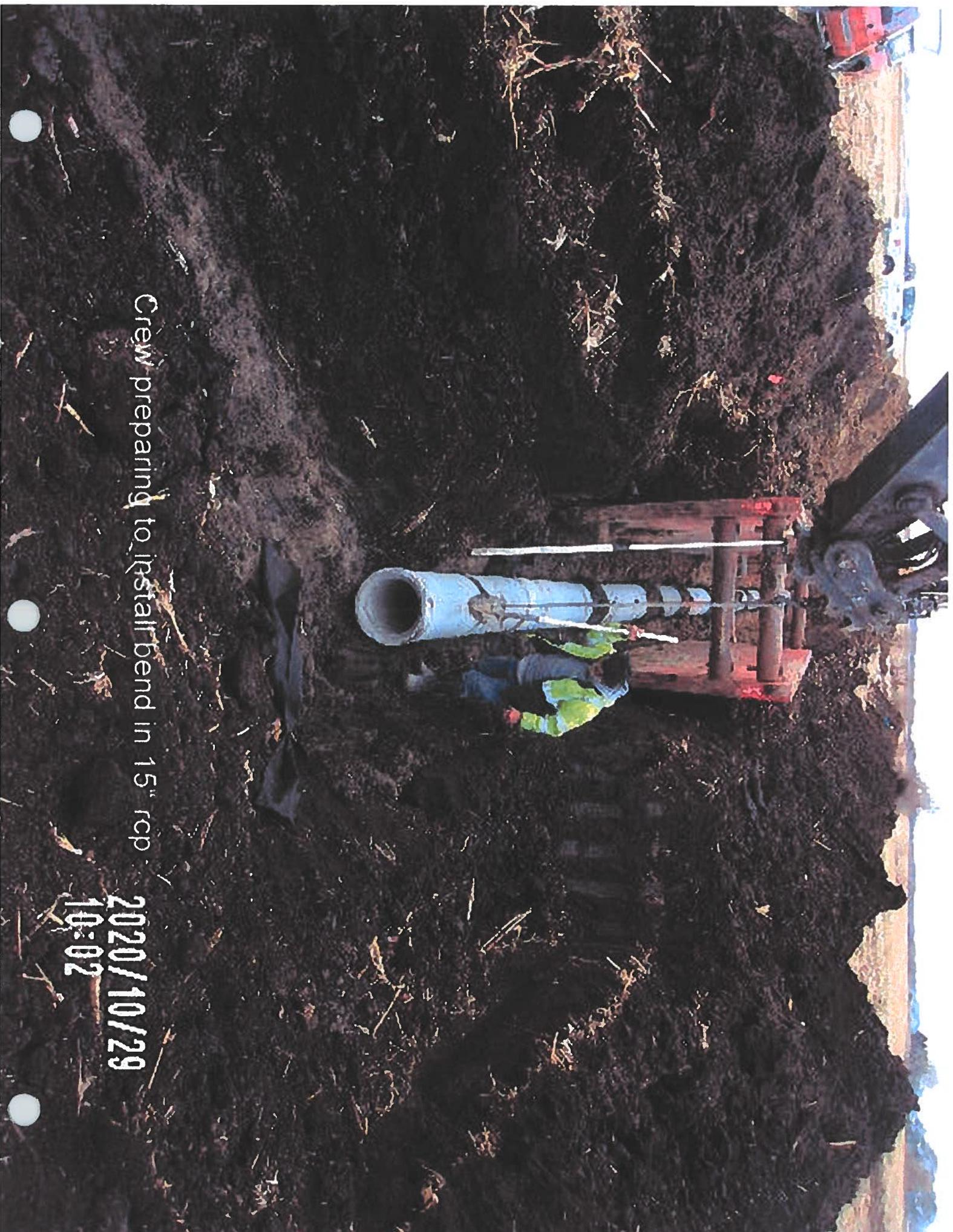
Bend cut and installed in 15" rcp
